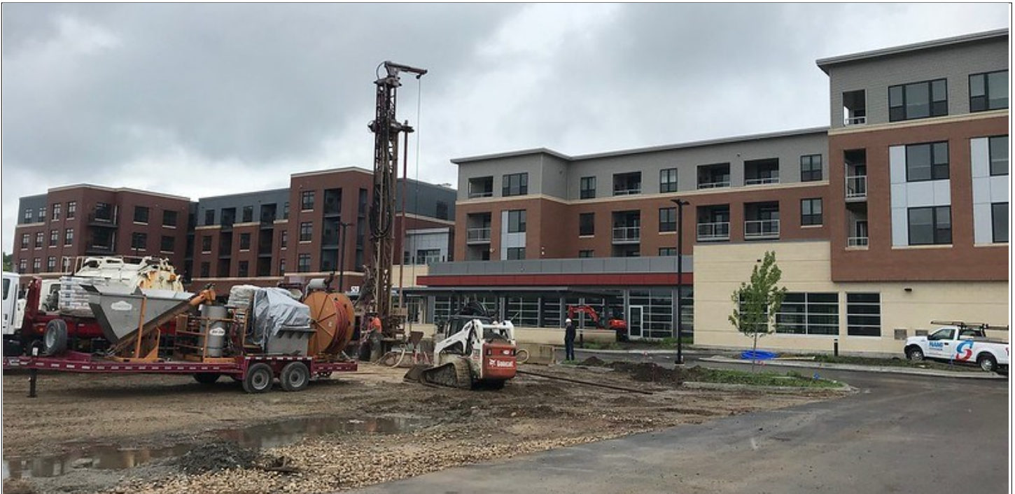
Construction on the new Royster development continues at a steady pace.
