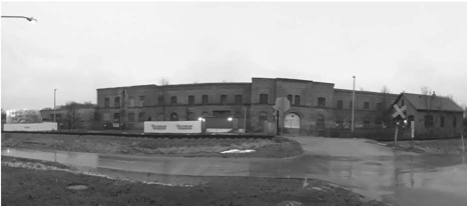
Renovation is underway at Garver Feed Mill!
