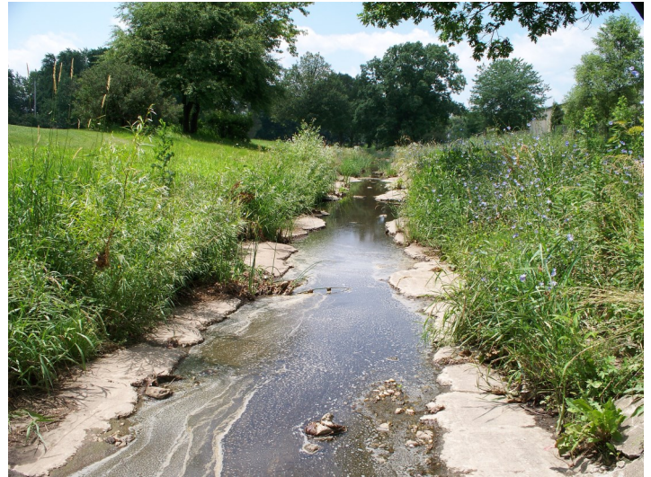
This picture above taken in July of this year is a section of the Eastmorland Park drainage ditch that runs east to west behind Woodman's Grocery. It shows how badly the concrete is broken and the water it is holding going nowhere.
