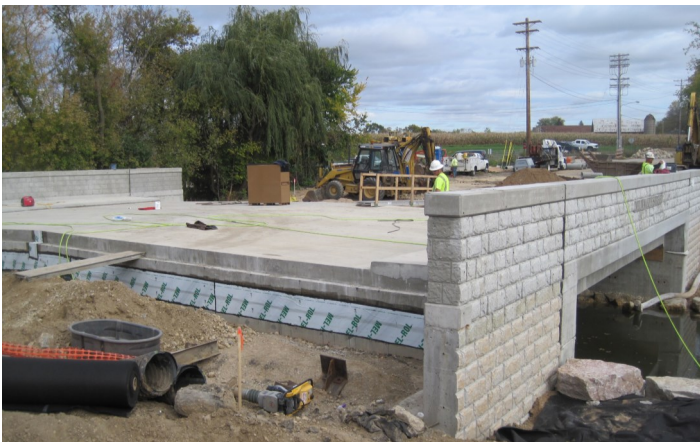
A view of the Milwaukee Street Bridge as of October 13, 2015. It would have been nice to show a picture of the completed bridge, but it is scheduled to be completed around the middle of November, and it will be a vast improvement over the old bridge.
